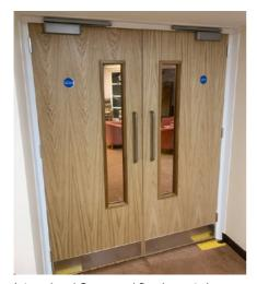
Internal and Communal fire doorsets have an important function to protect escape routes from the effects of fire so occupants can reach means of escape.
